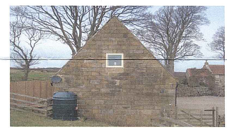
Photo of South Elevation
