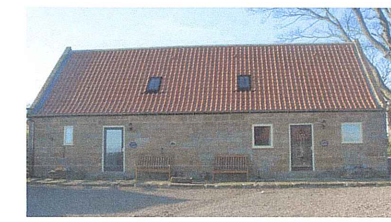
Photo of East Elevation
