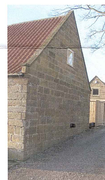
Photo of North Elevation
