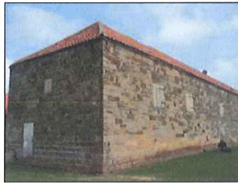
Photo 2: Granary north & west elevations
