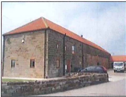
Photo 1: Granary eastern elevation
