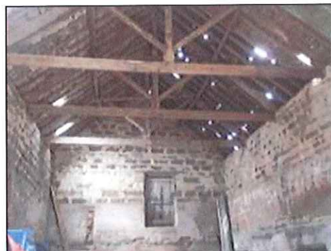
Photo 4: Lath / felt lined roof
