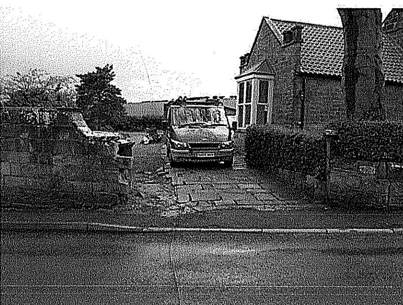
PHOTOGRAPH OF CURRENT SITE ENTRANCE: 26 APRIL 2012
