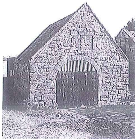
Inspiration for the proposed arch opening to the rear of Cottage 2: Cartshed at Beckside Farm, Danby
