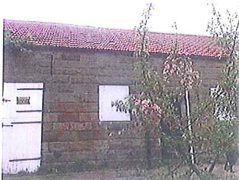
Road side elevation: Windows boarded up
