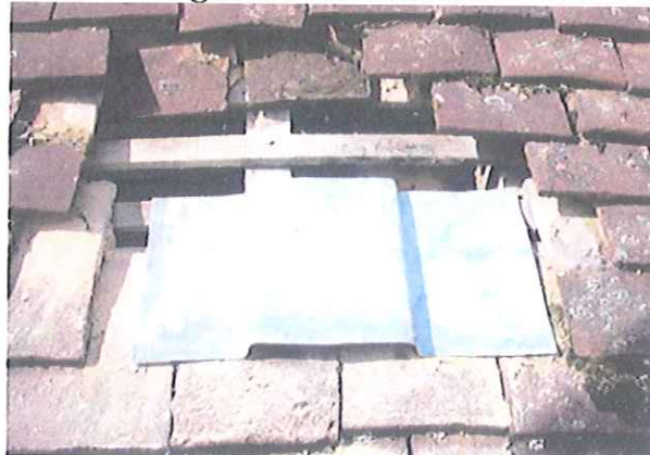
Figure 5b – Access slate.
