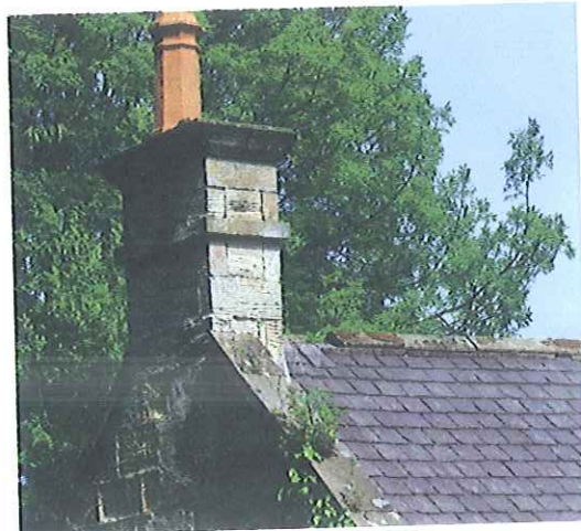
Chimney / Gable Coping / Ridge
