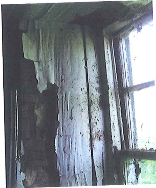
Window Reveal Lining Board
