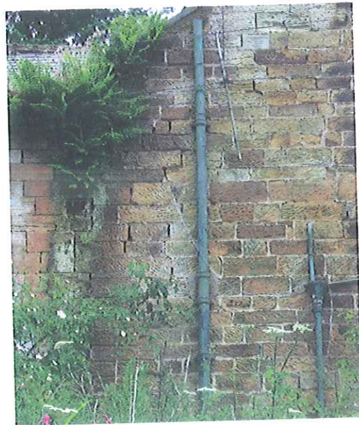
Wall junction between Main and Extension
