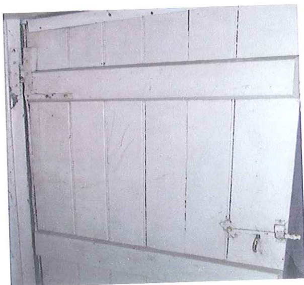
Boarded Door Hinge and Latch Detail
