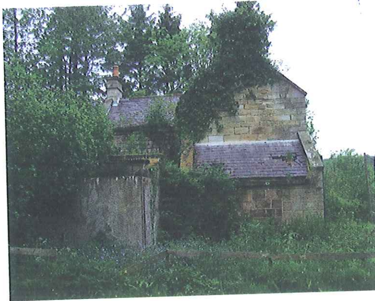
Derelict Garage in foreground obscured by fallen tree
