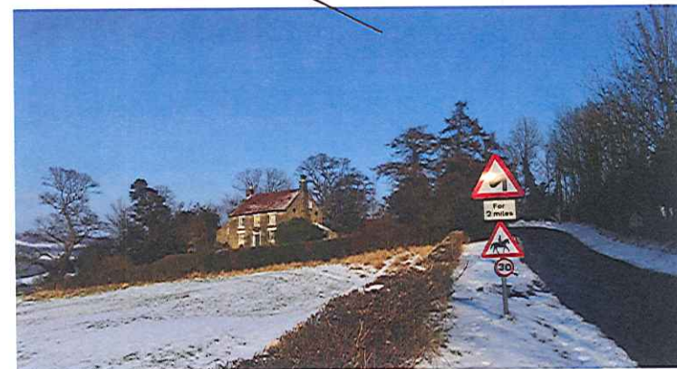
View looking from the South to 'Eskdale'
