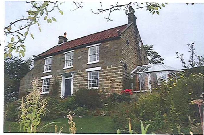
View from garden to front of 'Eskdale'
