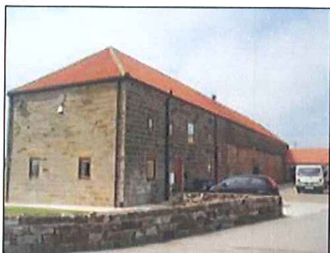
Photo 1: Granary eastern elevation
