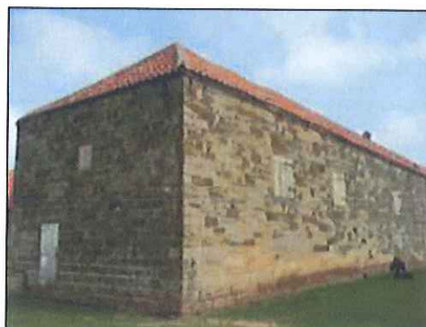
Photo 2: Granary north & west elevations
