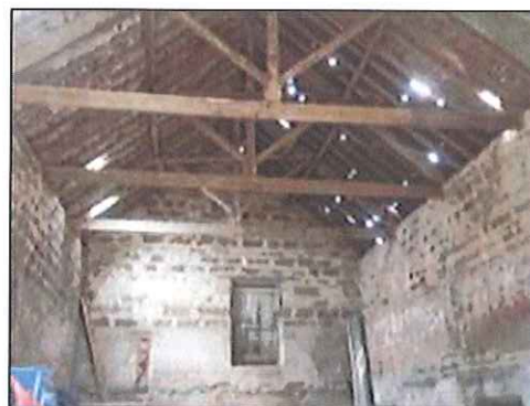
Photo 4: Lath / felt lined roof
