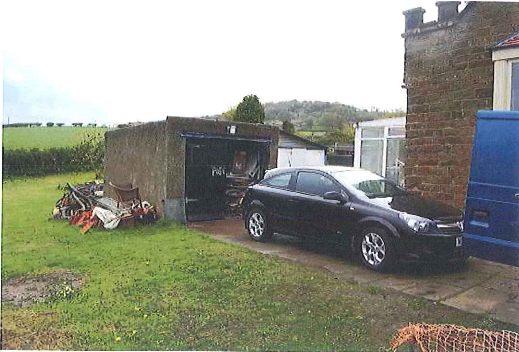
Views from within the site illustrating the existing garage structures to be removed.
