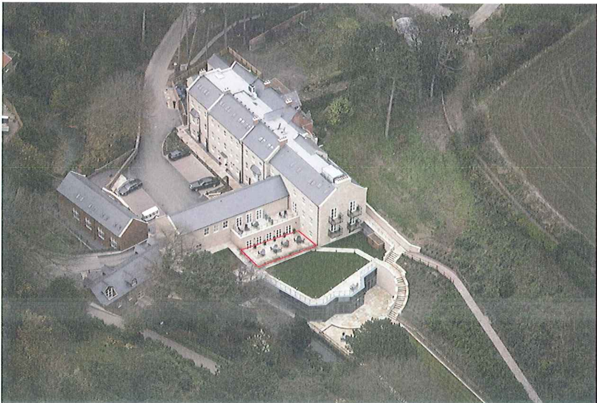
Raithwaite Hall as Existing. (Red line indicates the area of extension)
