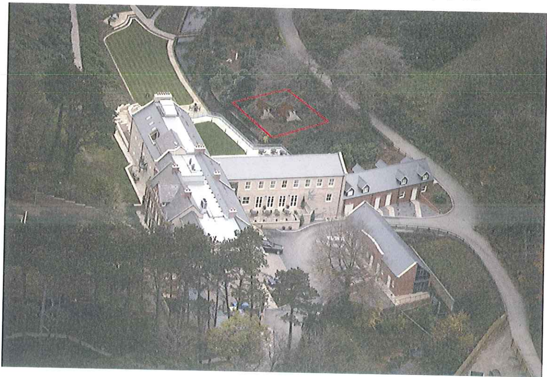
Raithwaite Hall as Proposed. (Red line indicates the location of sap pods)
