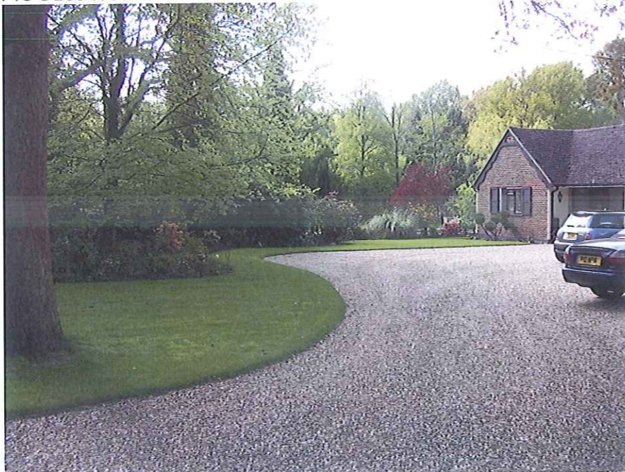
Photo 11 – Typical Gravel drive
