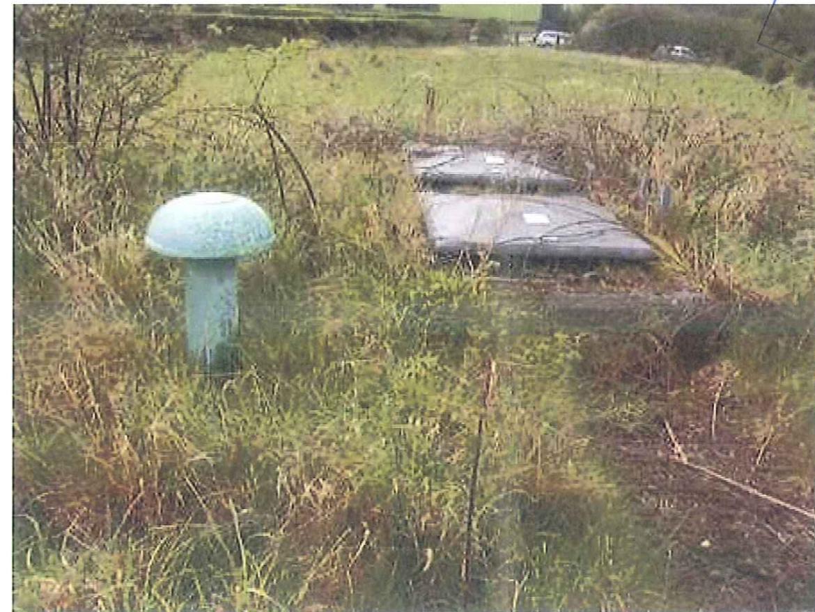
Photo 9 – top of reservoir structure
