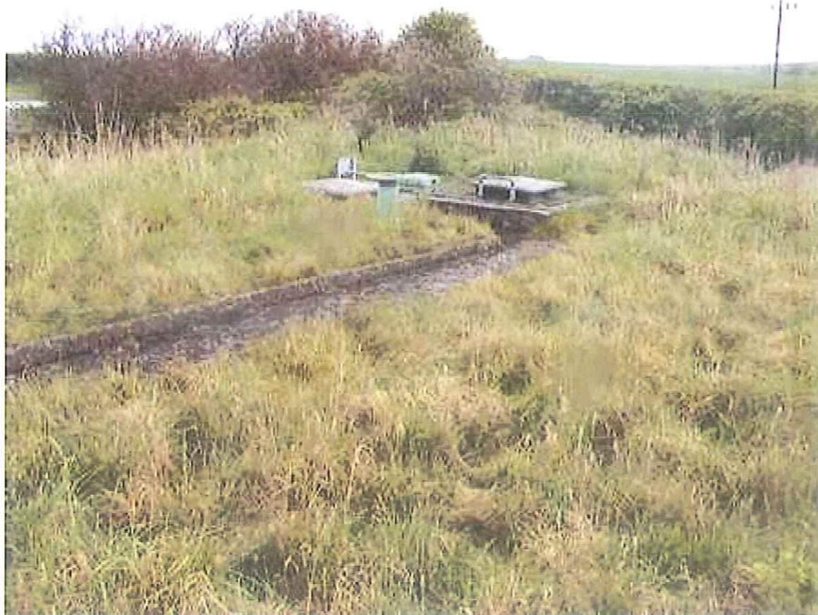
Photo 8 – top of reservoir structure
