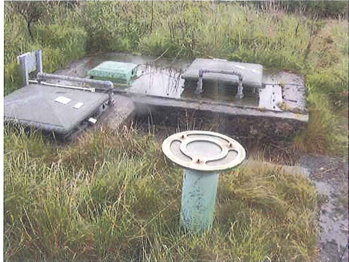
Photo 7 –top of reservoir structure
