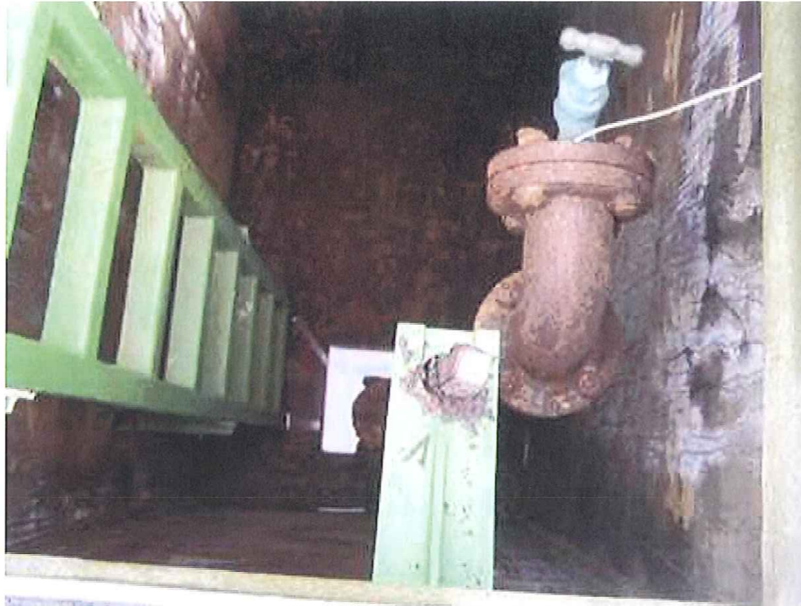
Photo 6 – Concrete Chamber in reservoir
