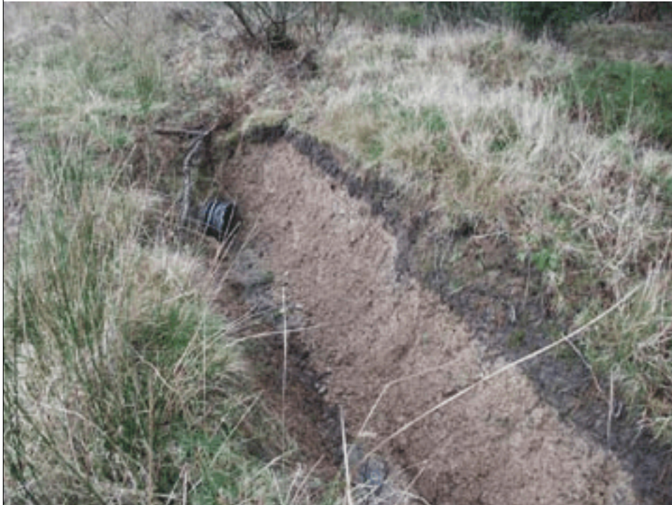
Fig 5 Drainage trench showing shallow soil horizons
