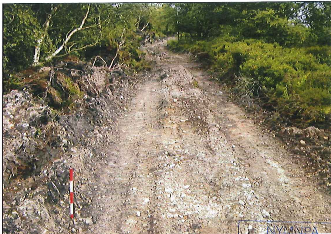
Plate1: The excavated track, facing west
