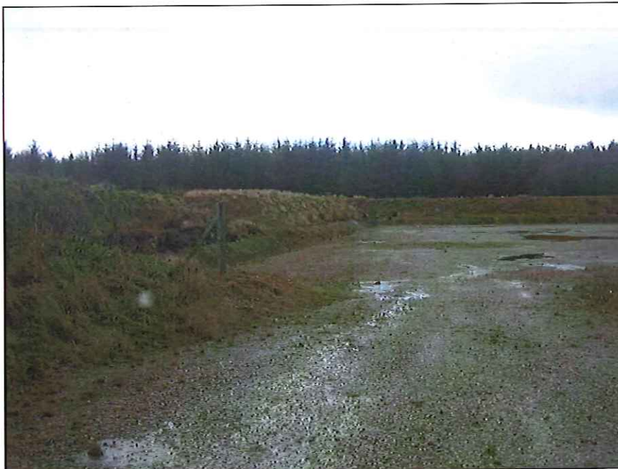
Photograph 2: Naturally re-colonised topsoil storage bund around site
