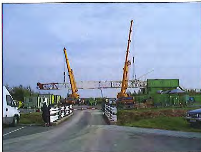
Figure 10. Rigging up Rig 40
