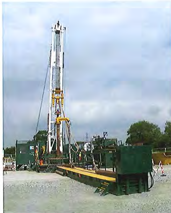
Figure 9. Drilling Rig Typically Used to Set the Conductor in the Cellar
