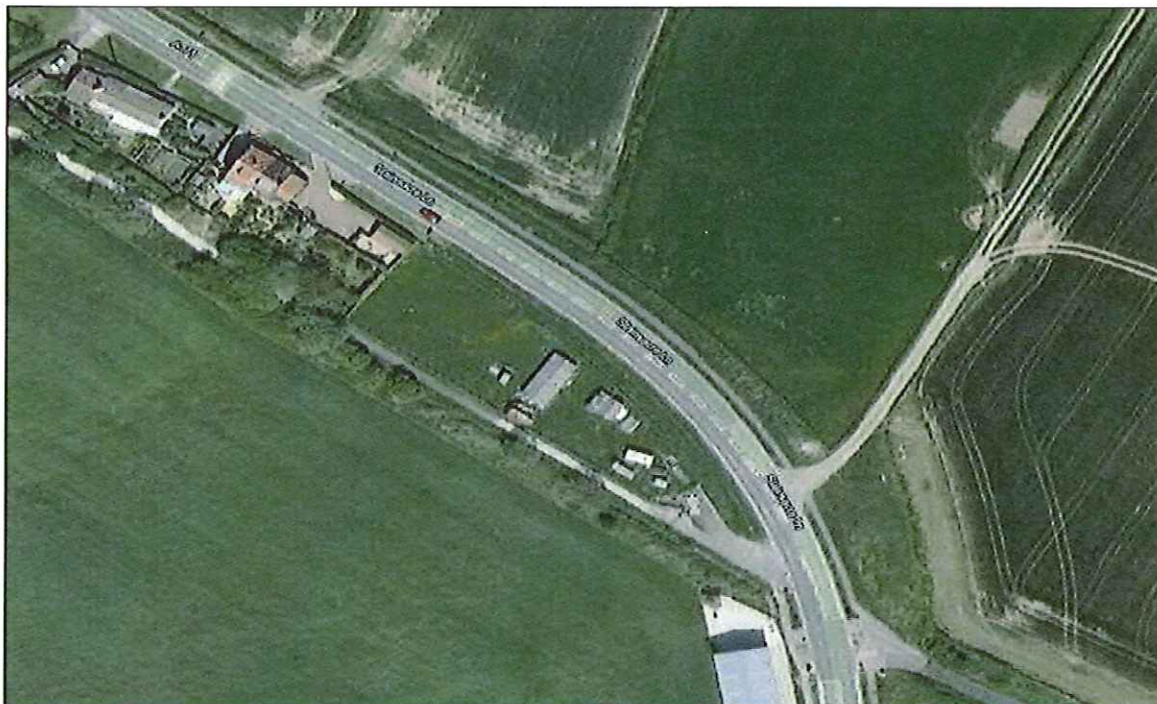
Photograph 2 - Aerial View showing previous Structures
