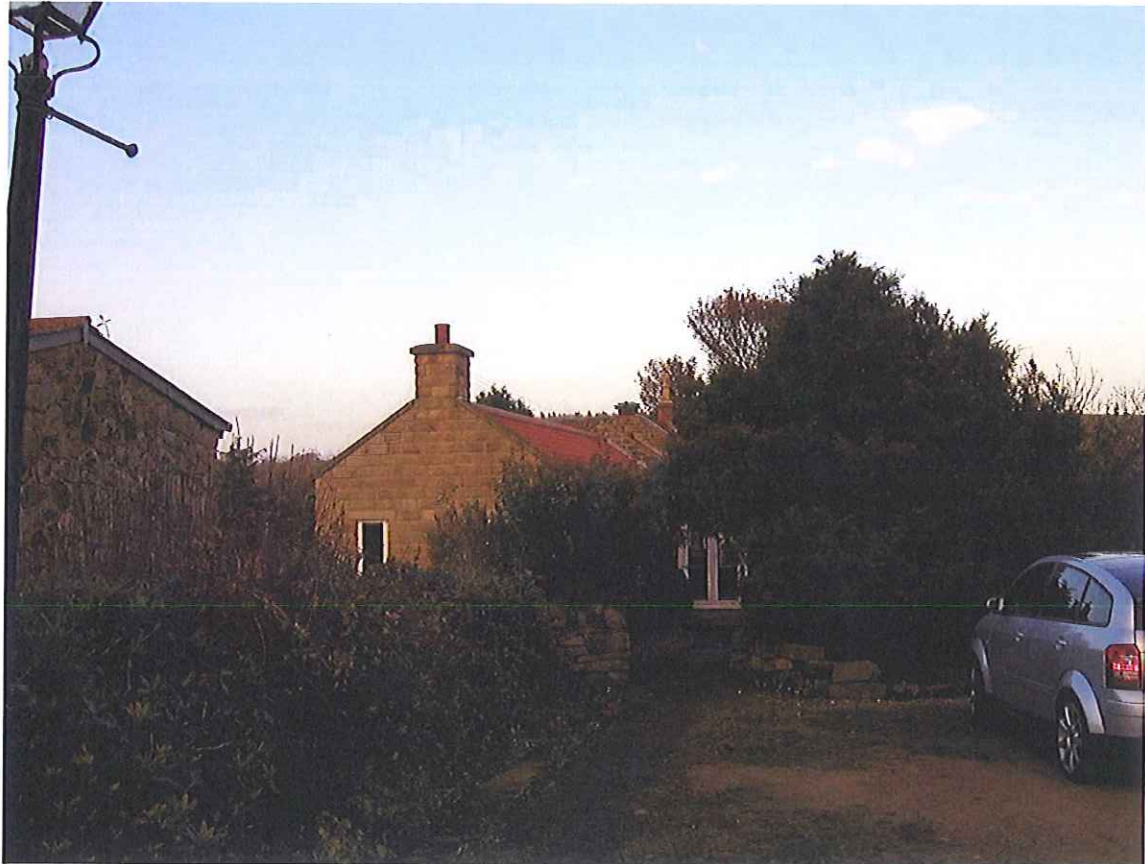
Fig.8 South-west gable end and parking area
