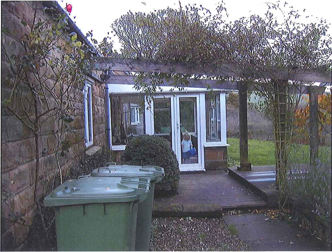
Fig.5 Entrance doors to the conservatory
