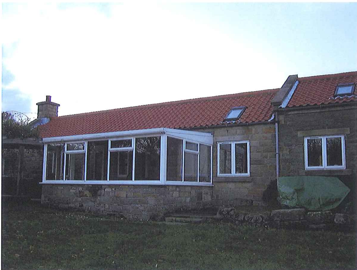
Fig.7 Part south-east elevation with conservatory and newest part of the house
