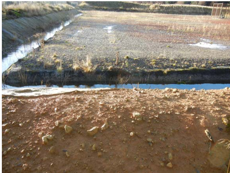
Photograph 15.1b. Ebberston 'A' Wellsite soil bund comprising of superficial material.
