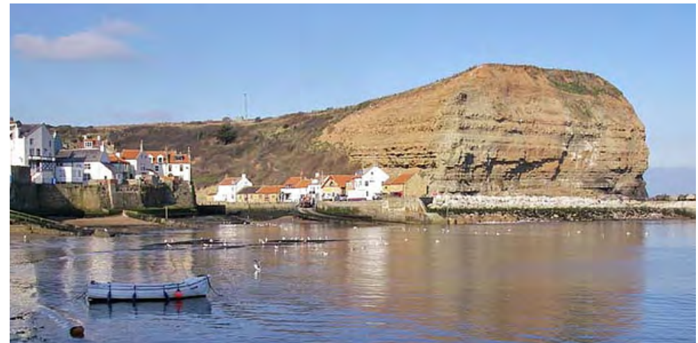
Coastal defences at larger settlements such as Staithes (above), Runswick, Whitby and Scarborough are currently managed to 'hold the line'
