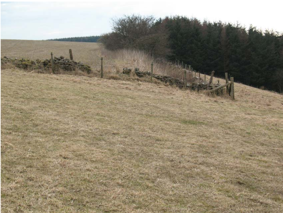
Plate 10: Ryedale Gas Project: view along the Givendale Lower Dike (MNY5454; SM35442) from the north where crossed by the pipeline corridor (11 March 2010)
