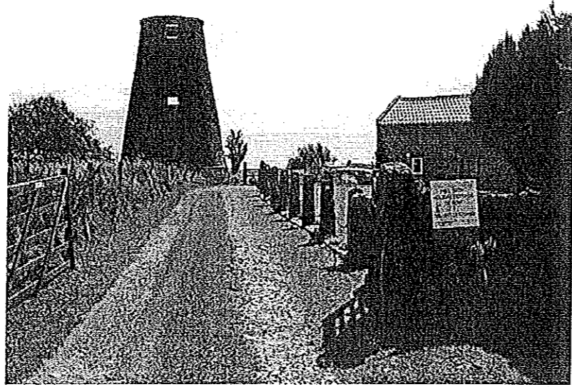
PRIVATE ACCESS ROAD FROM MAIN ROAD/ WEST VIEW
