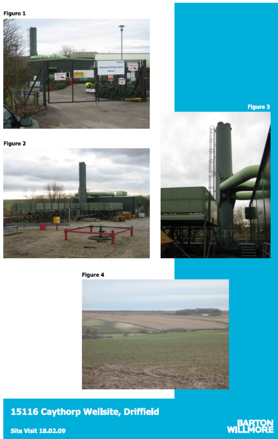
Figure 5.2 - Existing Electricity Turbine
