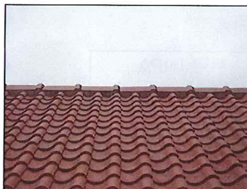
Photo 4: Sealed ridge tiles
