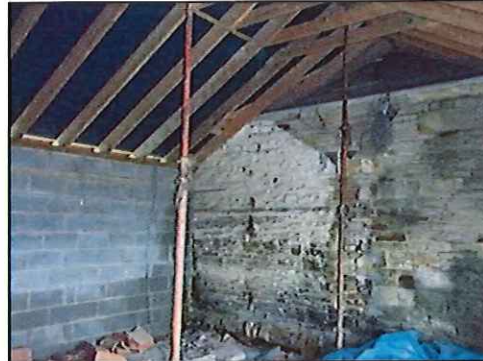
Photo 6: Stone wall at western end
