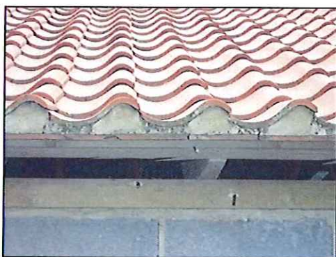
Photo 3: Sealed roof
