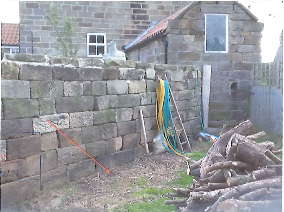
Location of oil tank will be minimum of 10cm under top of wall
