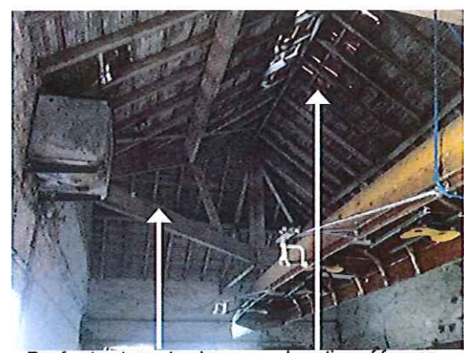
Roof structure to be retained and be visible within the conversion
