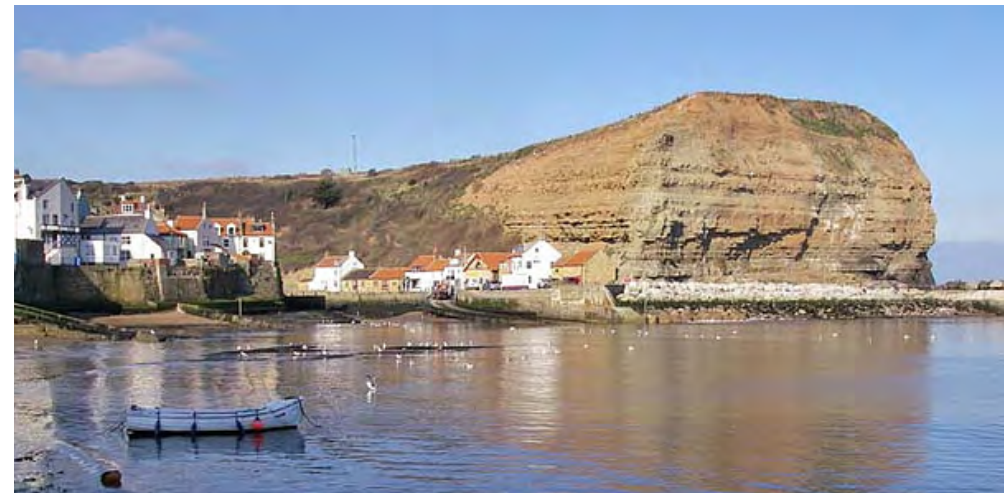
Coastal defences at larger settlements such as Staithes (above), Runswick, Whitby and Scarborough are currently managed to 'hold the line'
