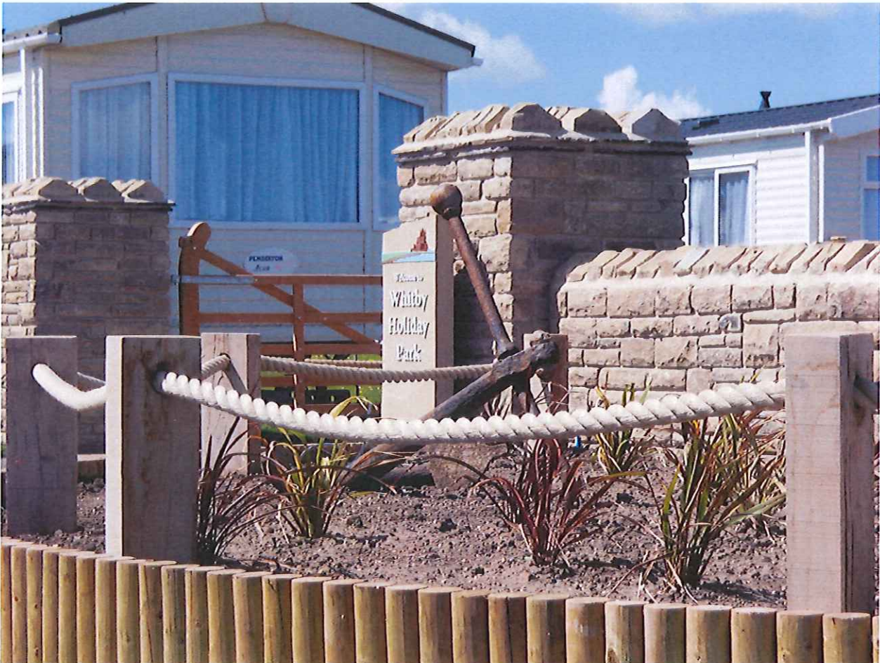
Figure 21. New entrance post construction, landscaping & planting to be completed.
