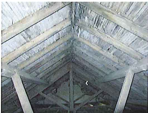
Fig 7 Roof void above stable (3).
