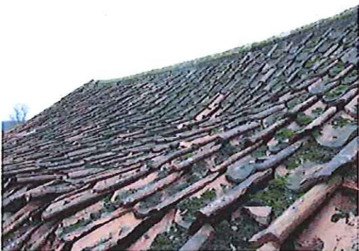
Fig 9 Roof of Building 5
