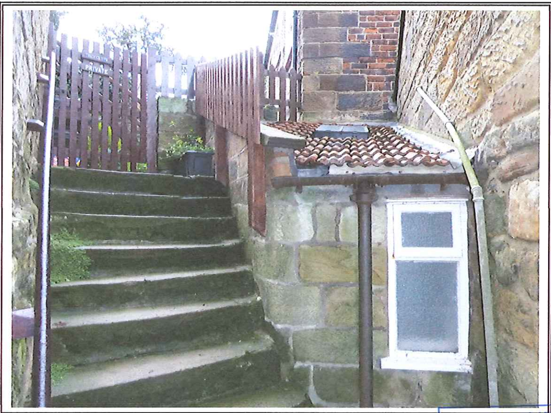
Photo 8 Roof after completion of works.
