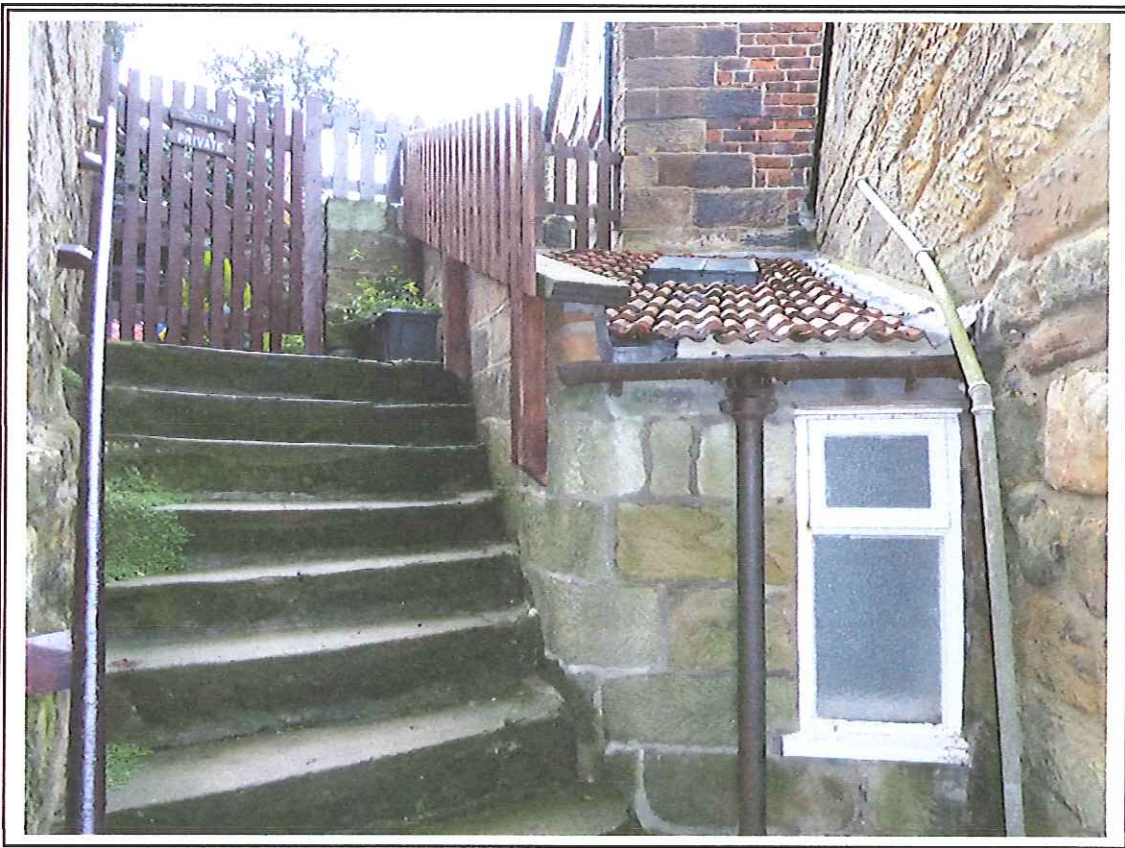
Photo 8 Roof after completion of works.
