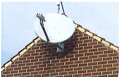
70cm solid dish mounted on 30cm J-Mount bracket on south elevation
