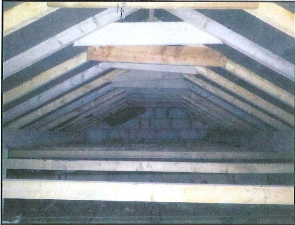
Photo 7: Inside Eastern roof Void.
