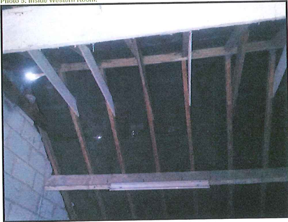
Photo 5: Inside Western Room.
