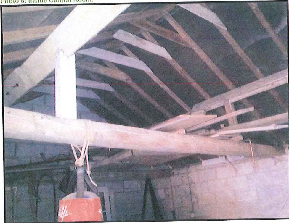
Photo 6: Inside Central Room.
