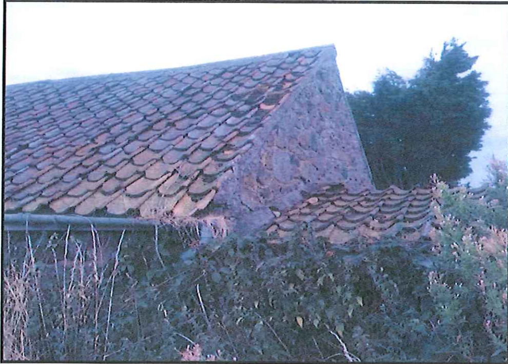
Photo 3: Western Gable with Adjoining Kennel.
