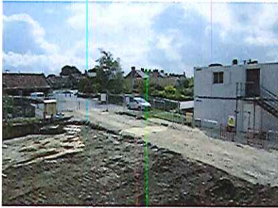
South east corner
