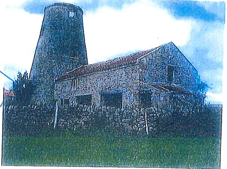
BEACON WINDMILL & BARN / VIEW FROM SOUTH EAST
