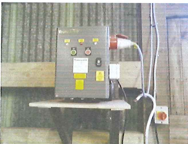
Phase converter, so I can have 3 phase machines which are easier to come by second-hand.
