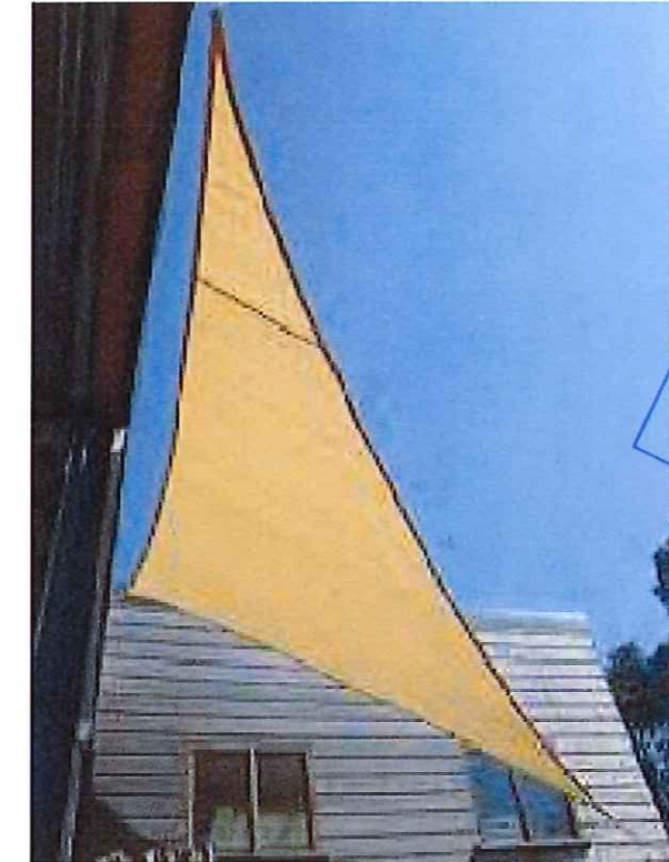
Sails attached back to building over entrance
