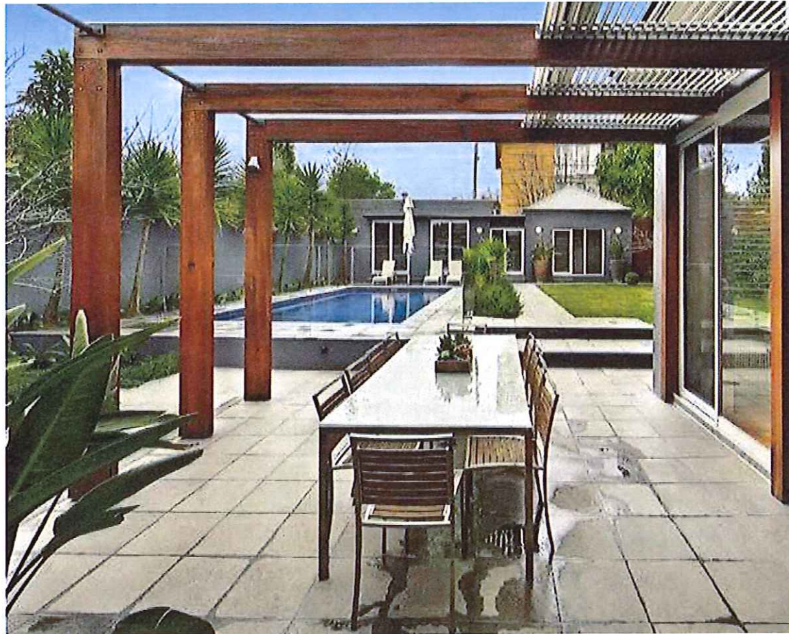
Pergola structure above decking to carry sails
