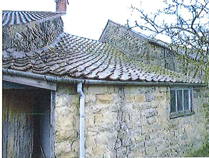
Plate 4 – Barn, west elevation.
