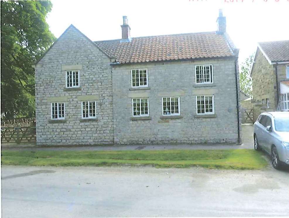
Existing Street Frontage elevation.
