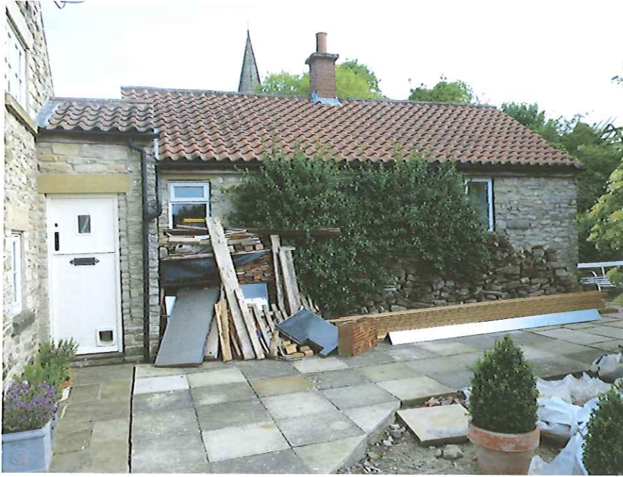
Later single storey extension – south elevation
