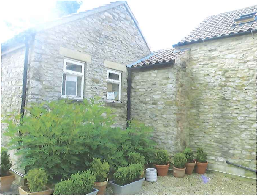
Later single storey extension – west elevation
