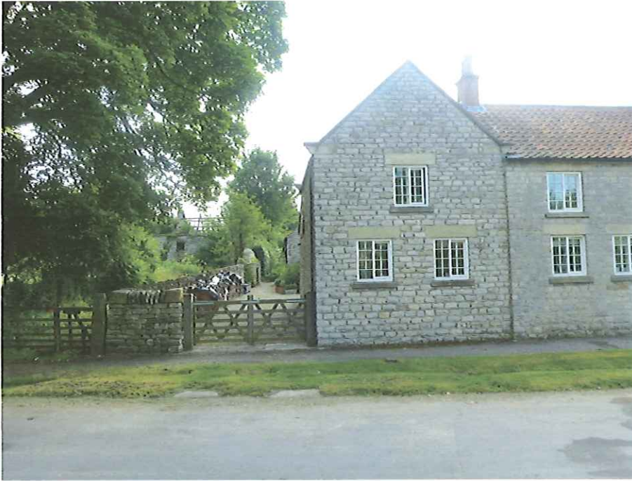
Existing vehicular access to the north.
