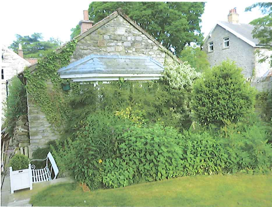
Later single storey extension – east elevation
