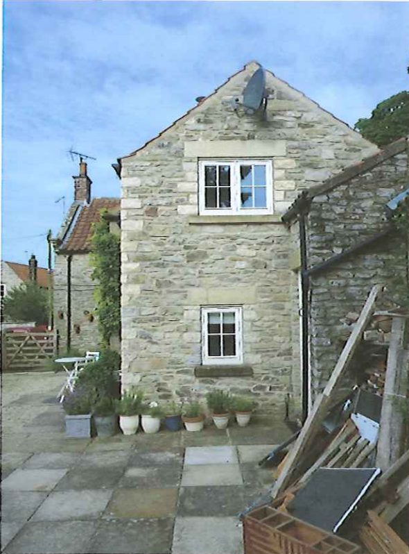
Main house – east elevation
