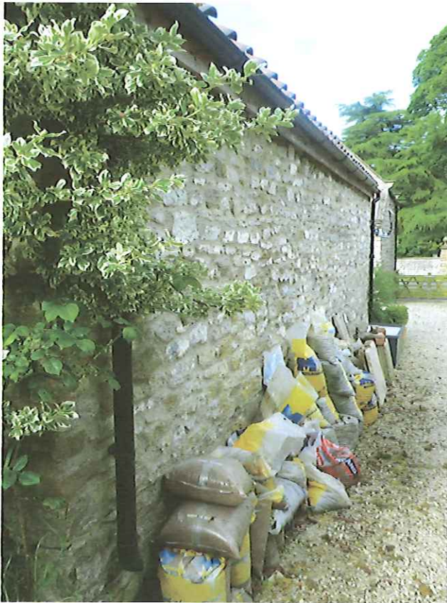
Later single storey extension – north elevation
