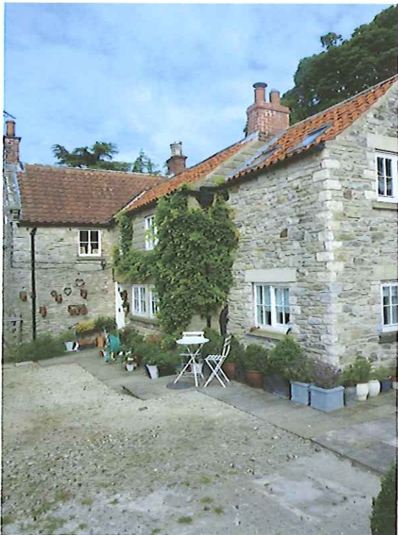
Main house – south elevation
