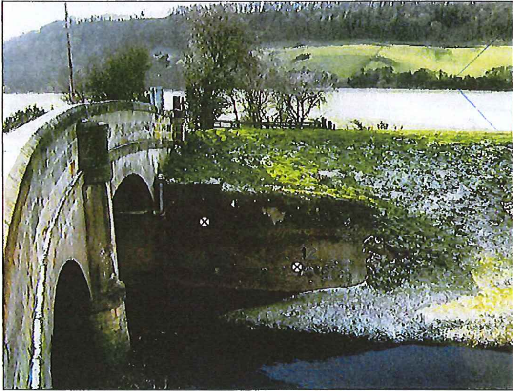
Photograph 5: South west wing wall. Cores required in indicative locations as shown.
