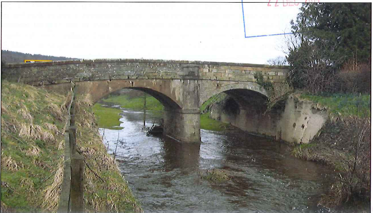
Mowthorp Bridge - Eastern Downstream Elevation
