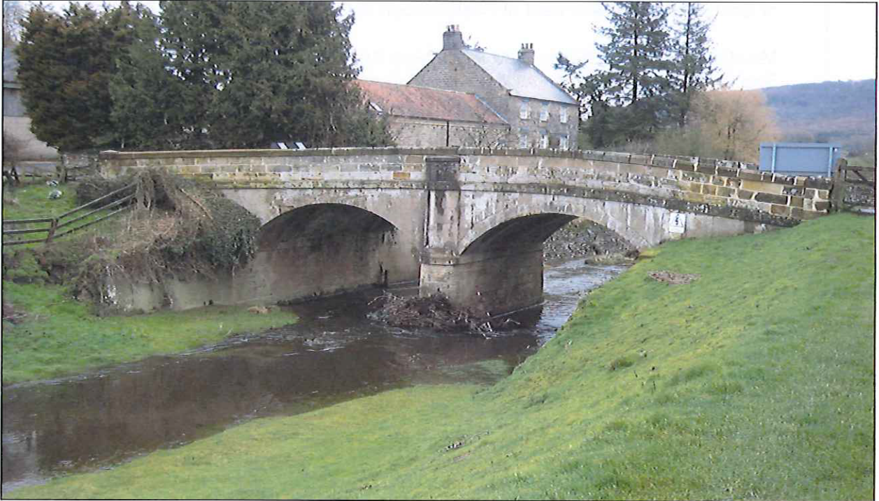
Mowthorp Bridge - Western Upstream Elevation
