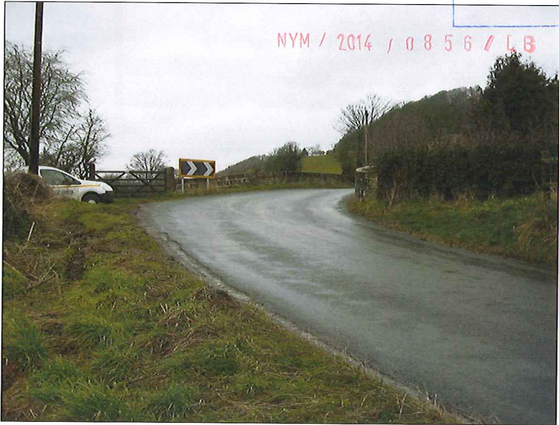
Photograph 1: Approach to bridge from south. Note sharp right hand bend on approach.
