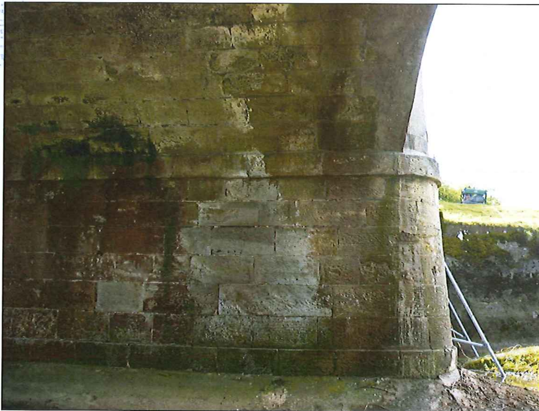
Photograph 34: Concrete widening #6 to western upstream side of north span.
