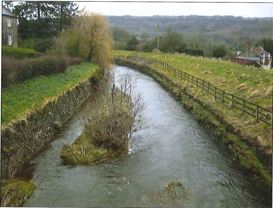
Photograph 6: View from bridge looking downstream to east.
