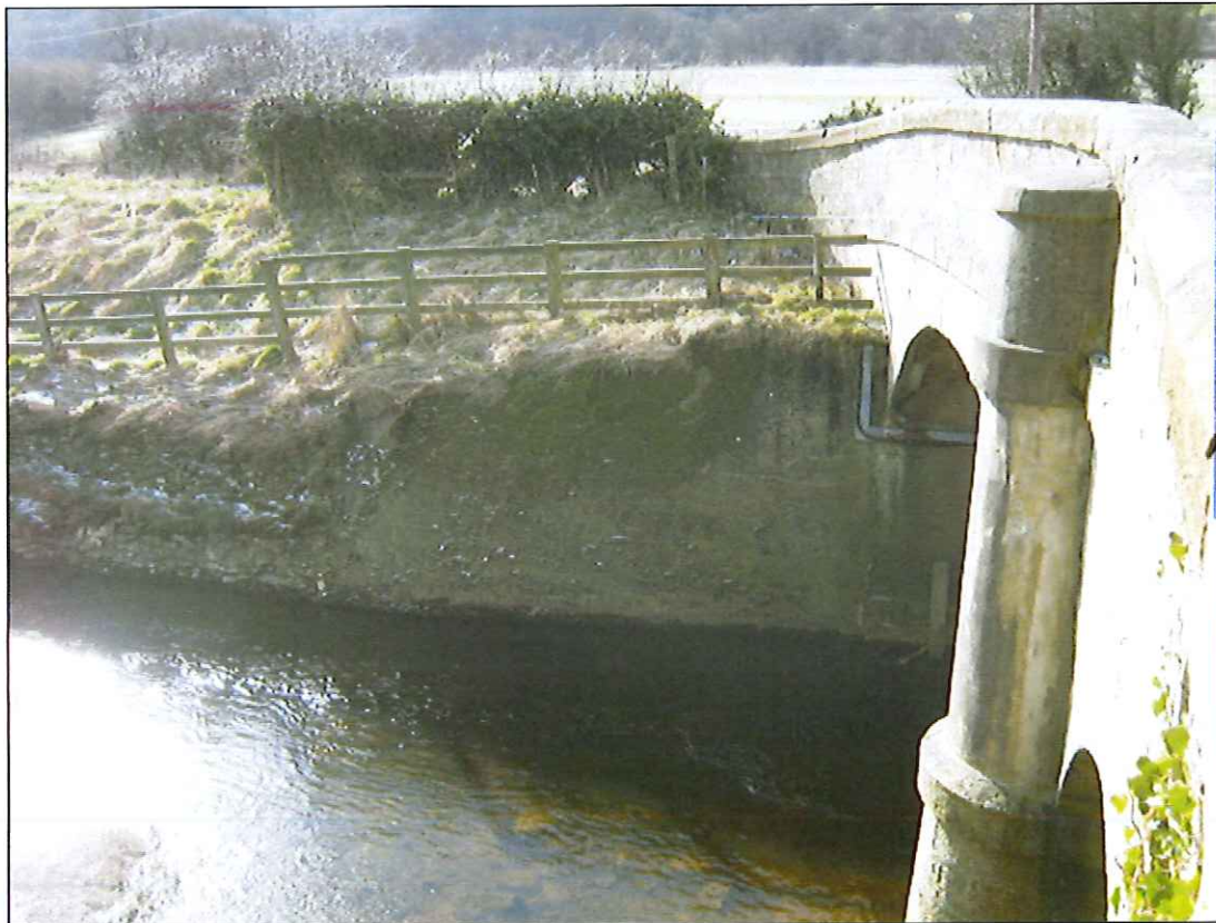
Photograph 16: South east wing wall constructed of rendered mass concrete.
