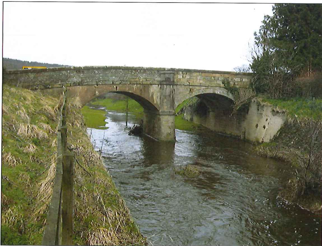
Photograph 10: Eastern downstream elevation.
