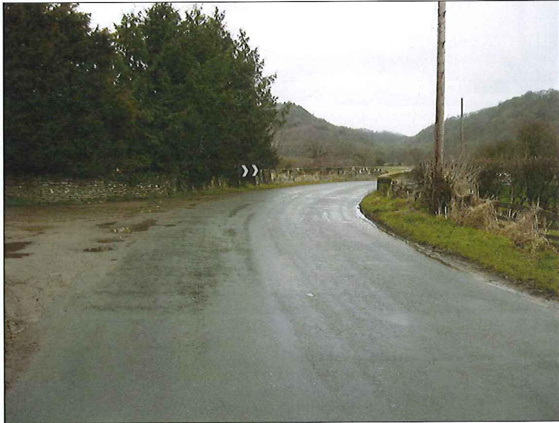
Photograph 3: Approach to bridge from north. Note sharp right hand bend on approach.
