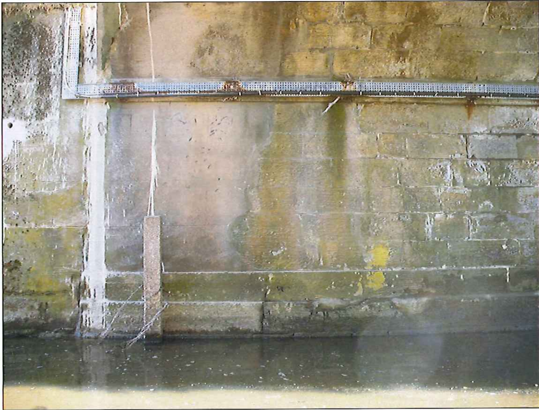
Photograph 23: South abutment, concrete widening #1 to eastern downstream side of south span.
