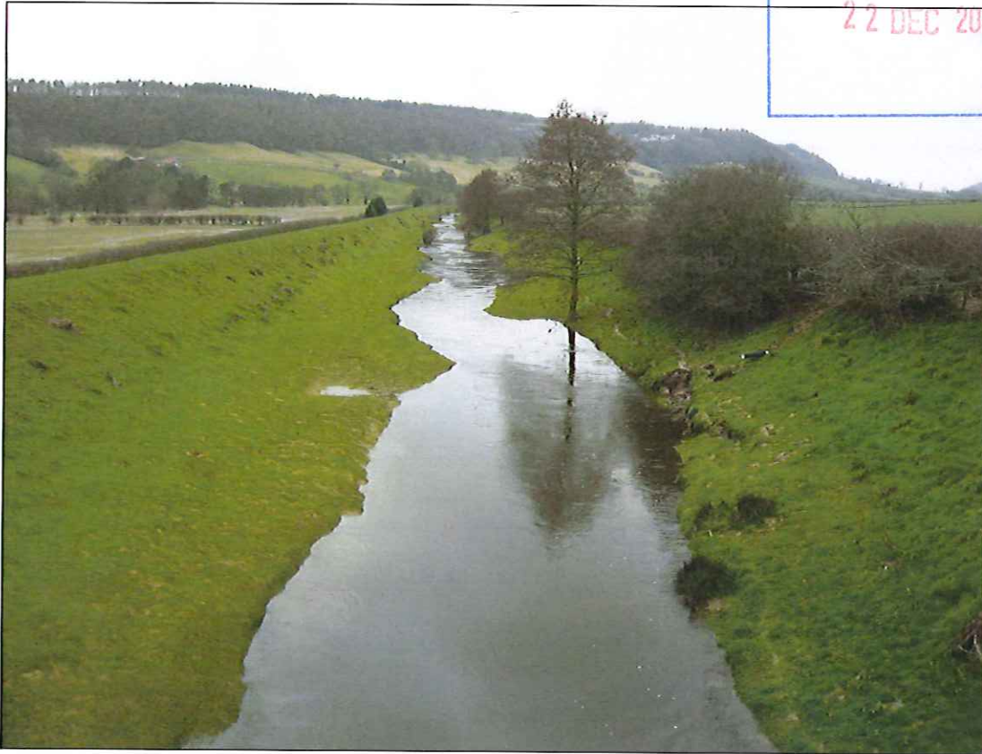
Photograph 5: View from bridge looking upstream to west.
