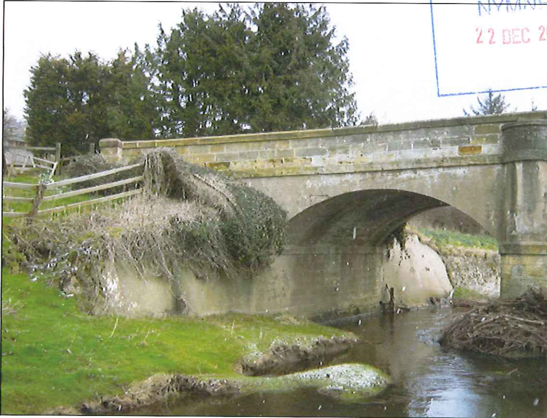
Photograph 17: North abutment and wing walls.
