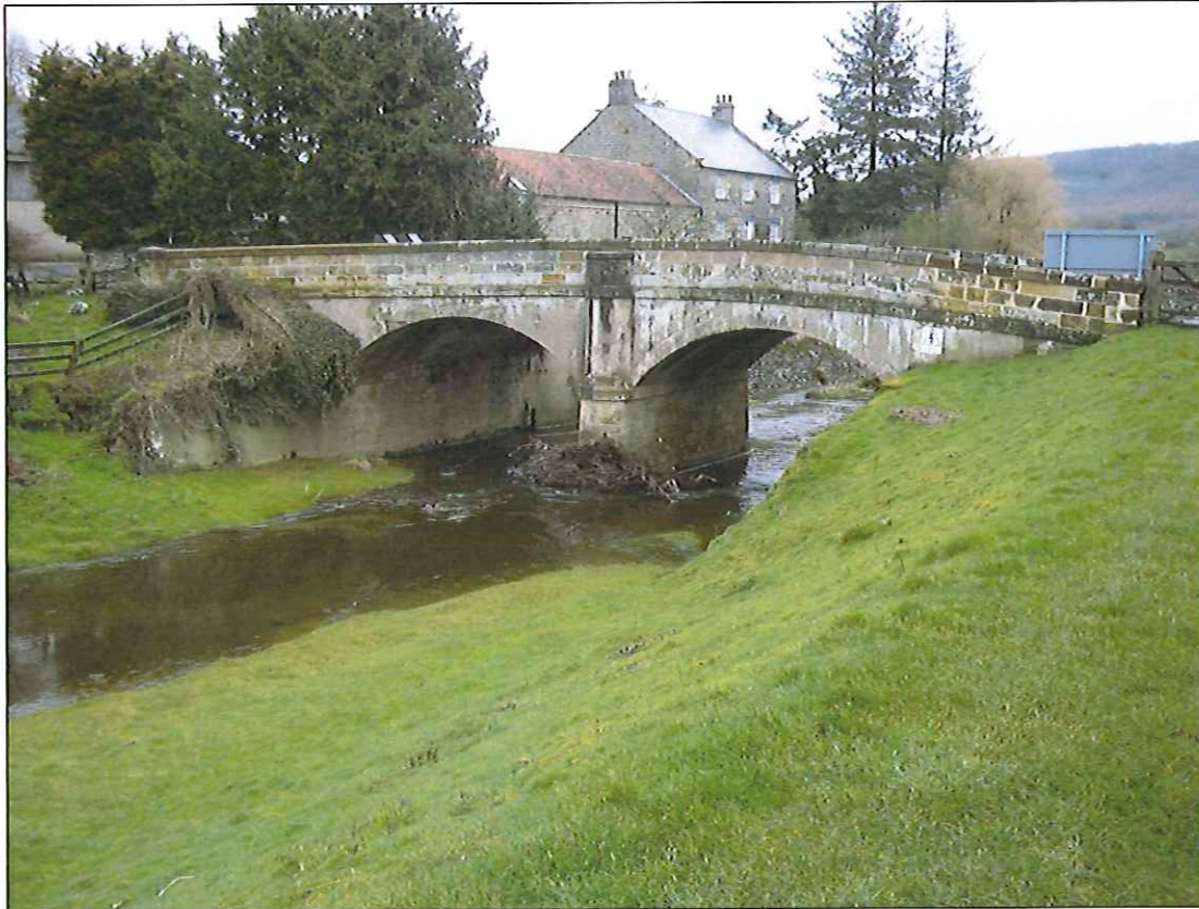
Photograph 7: West upstream elevation.
