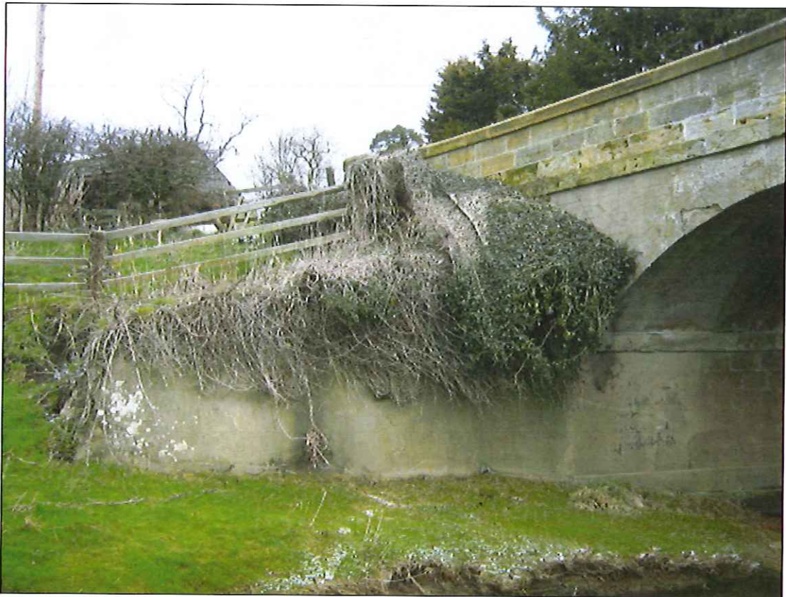
Photograph 18: North west wing wall constructed of rendered mass concrete.
