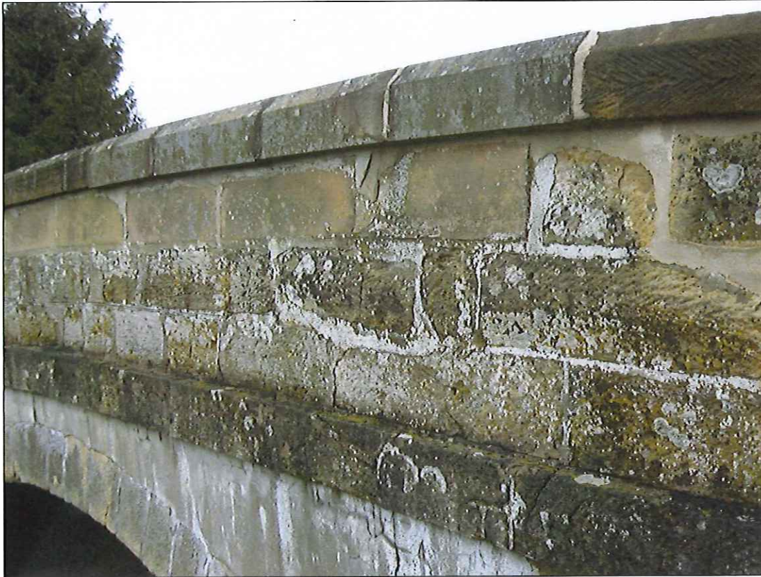
Photograph 35: Typical detail of outside face of parapet.
