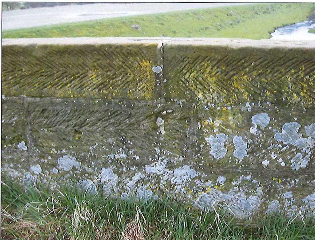
Photograph 38: Typical detail of inside face of parapet.
