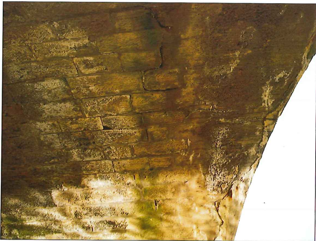
Photograph 26: Concrete widening #4 to eastern downstream side of south span. Note circumferential cracking.
