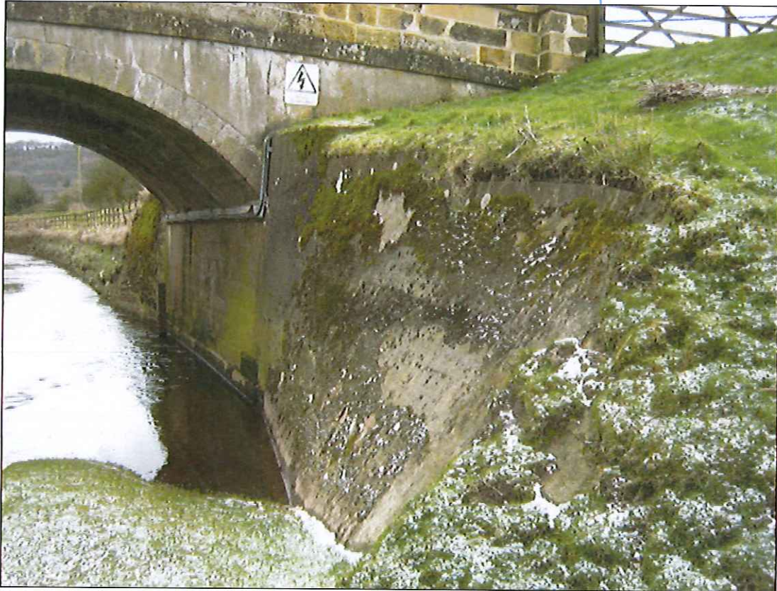
Photograph 13: South abutment and mass concrete south west wing wall.
