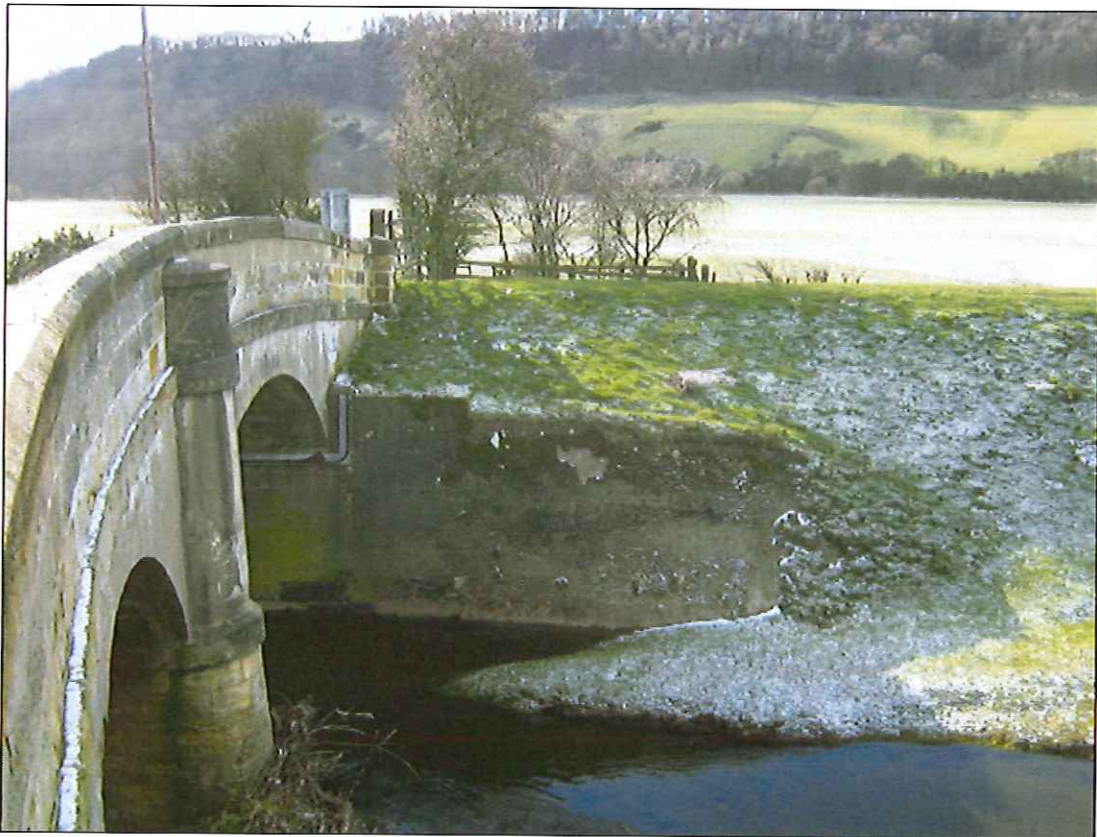
Photograph 14: South west wing wall constructed of rendered mass concrete.
