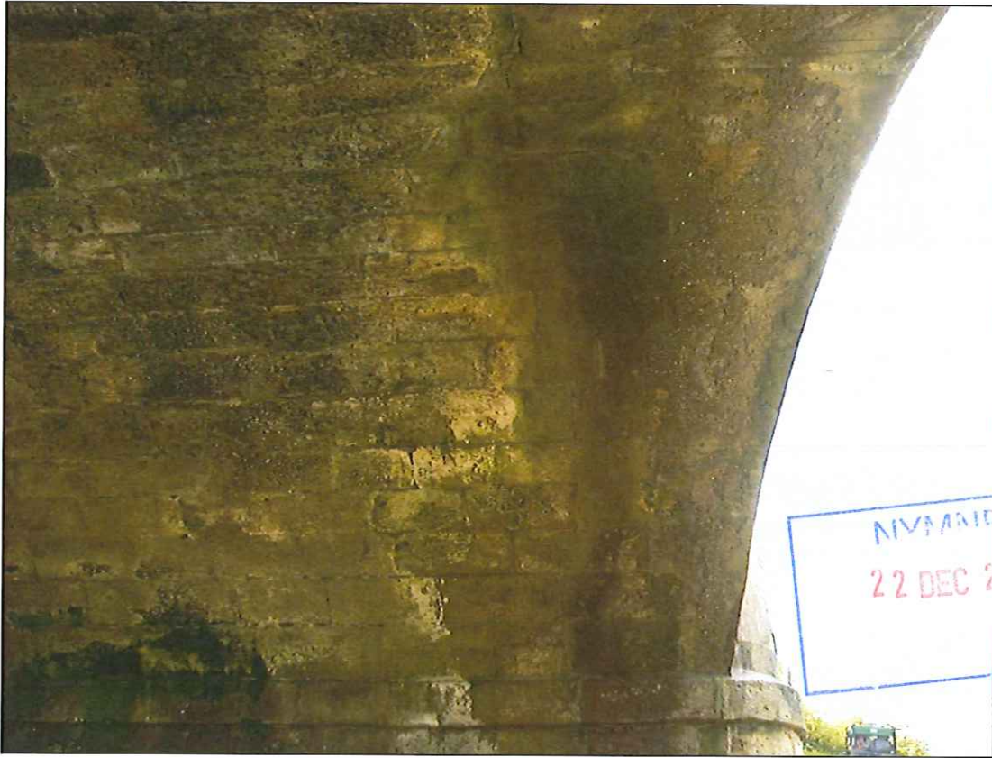
Photograph 33: Concrete widening #5 to western upstream side of north span.
