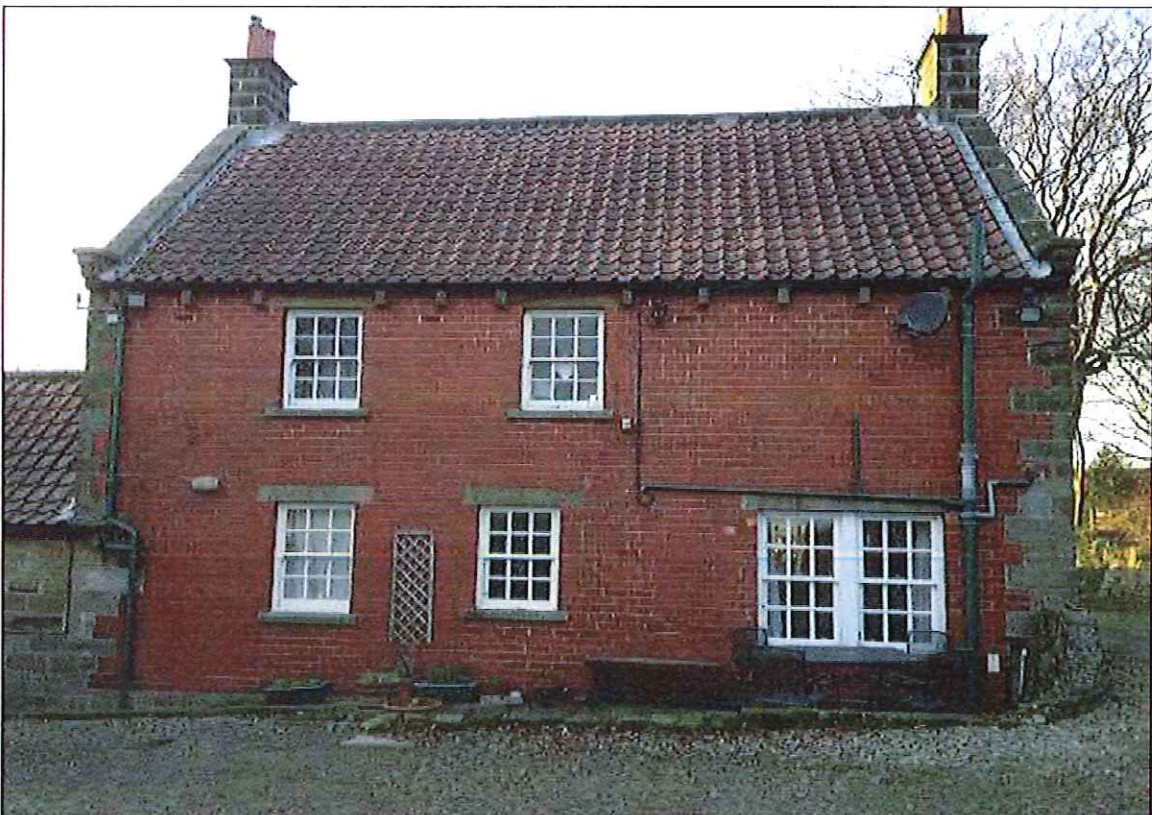
PHOTOGRAPH 1 Existing Rear Elevation
