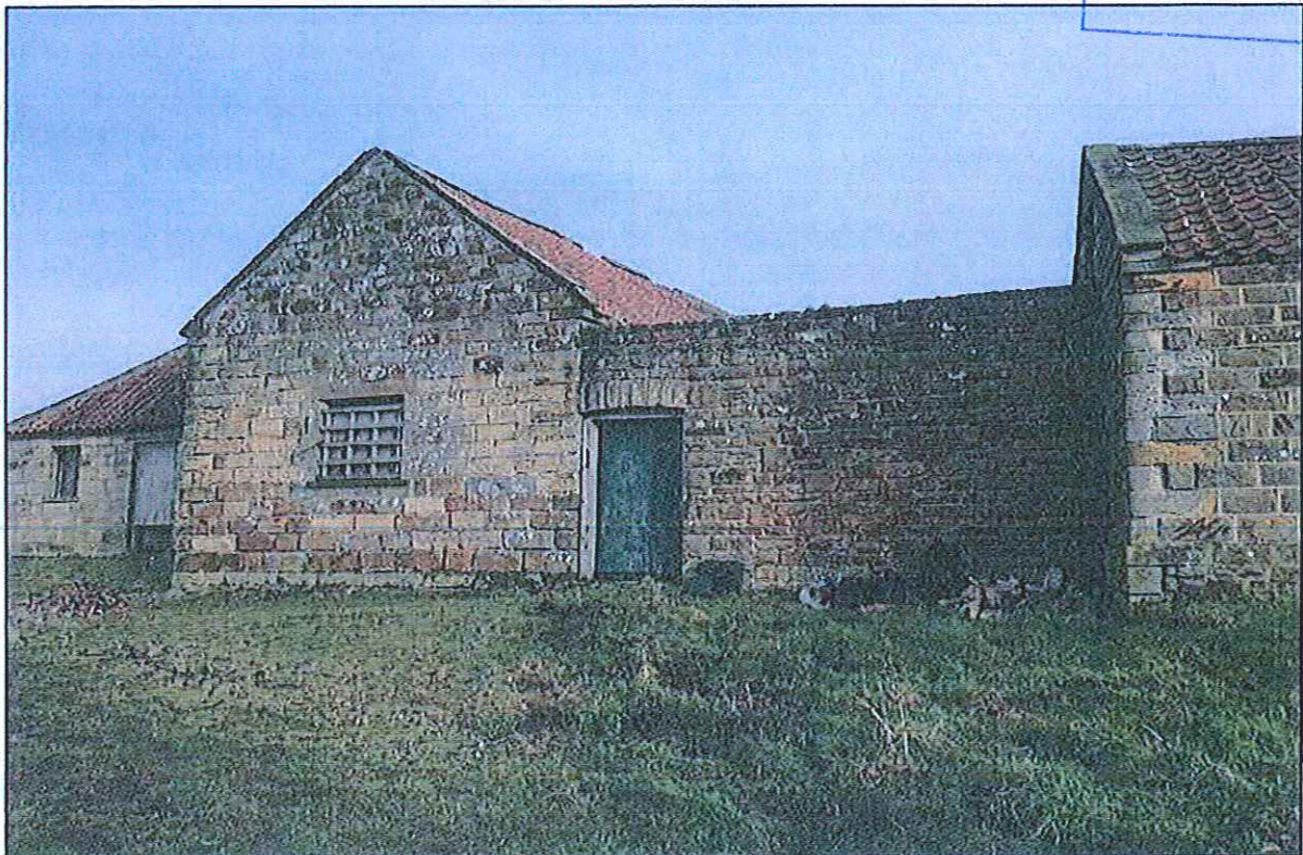
PHOTOGRAPH 8 Building A West Gable
