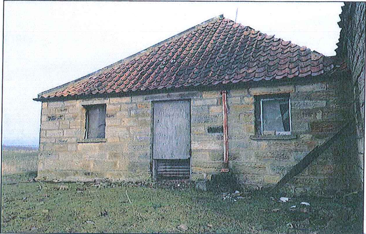
PHOTOGRAPH 9 Horse Engine Shed Building a West
