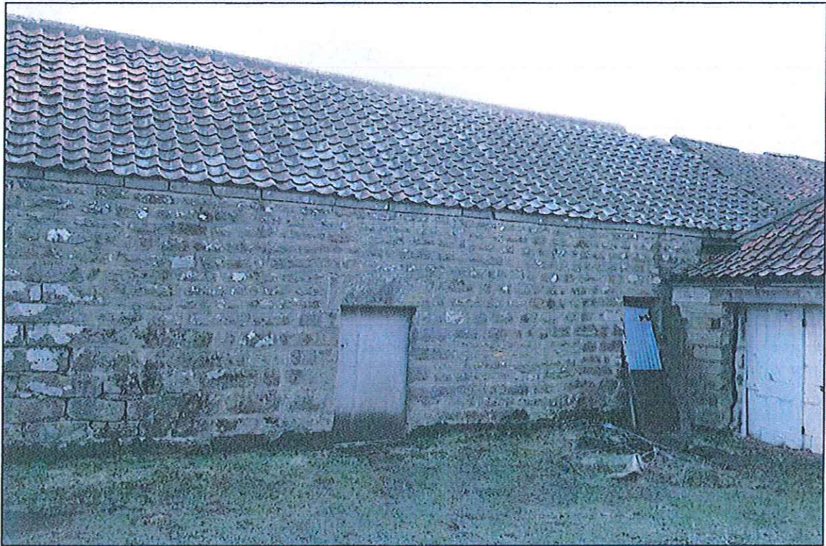
PHOTOGRAPH 11 Building A Rear/North
