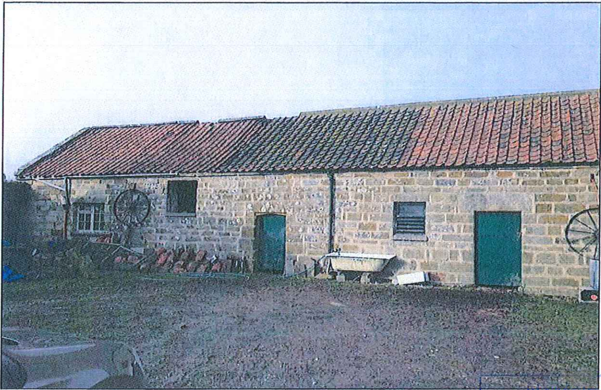
PHOTOGRAPH 3 Building A South Elevation
