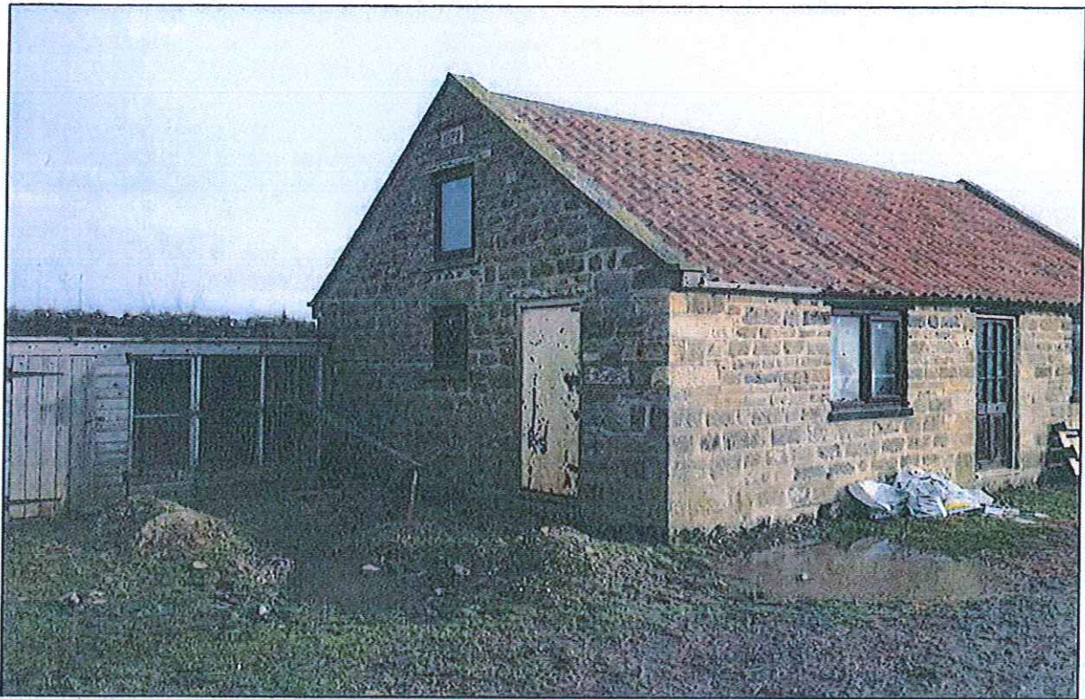
PHOTOGRAPH 5 Building C Side/North
