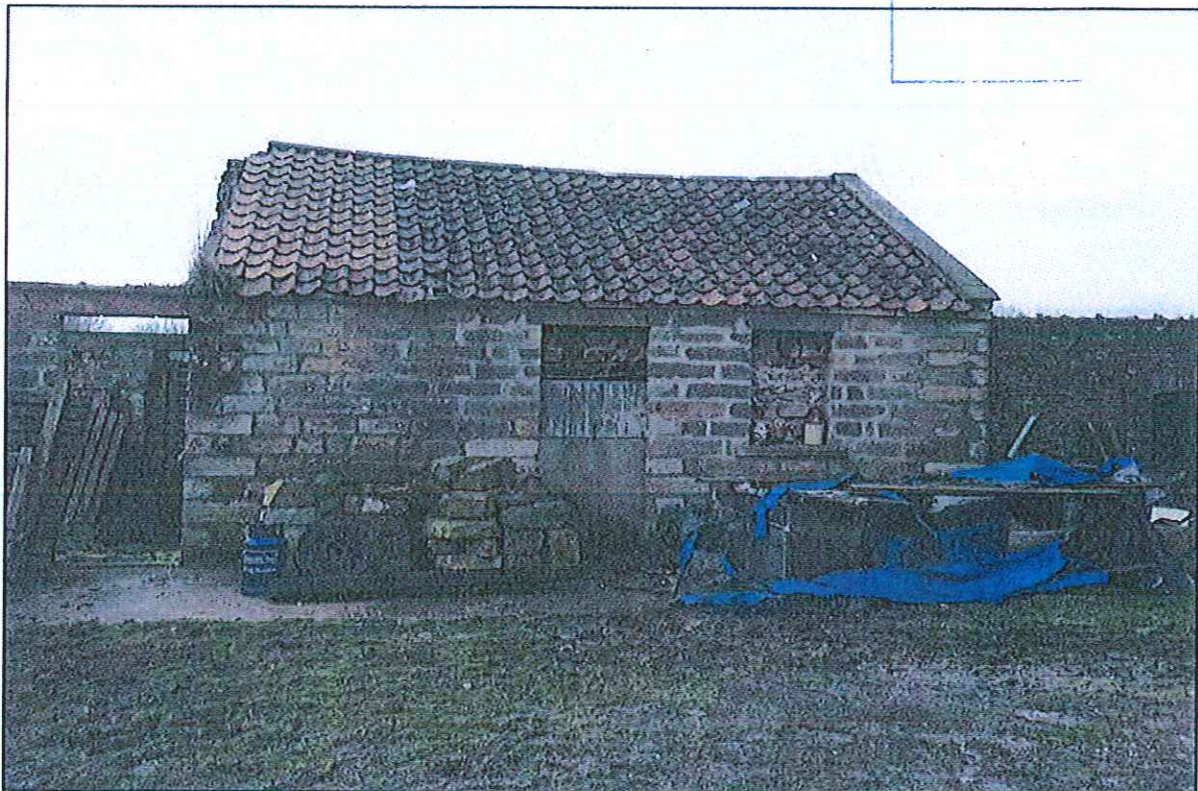
PHOTOGRAPH 6 Building B Front/East
