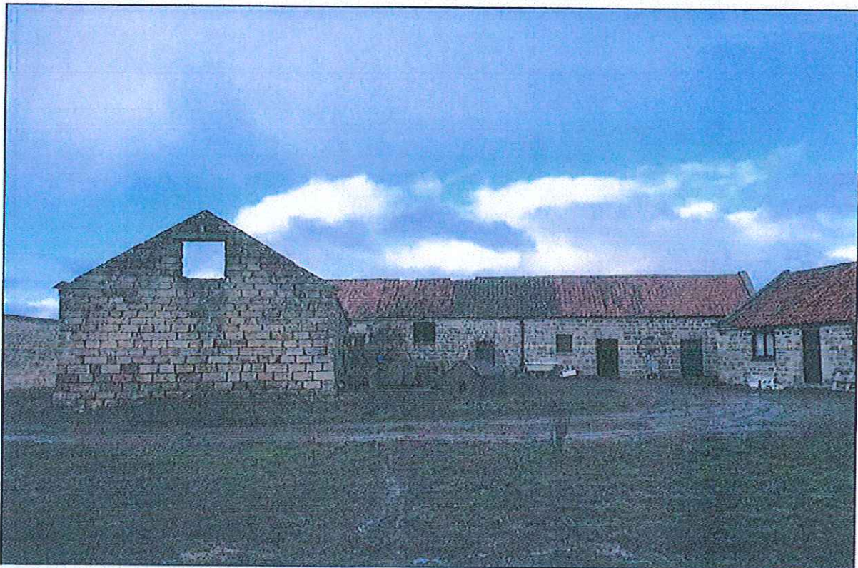
PHOTOGRAPH 2 Gable of Building B and Building A to Rear
