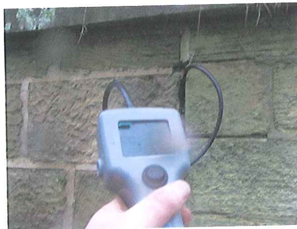
East elevation wall
