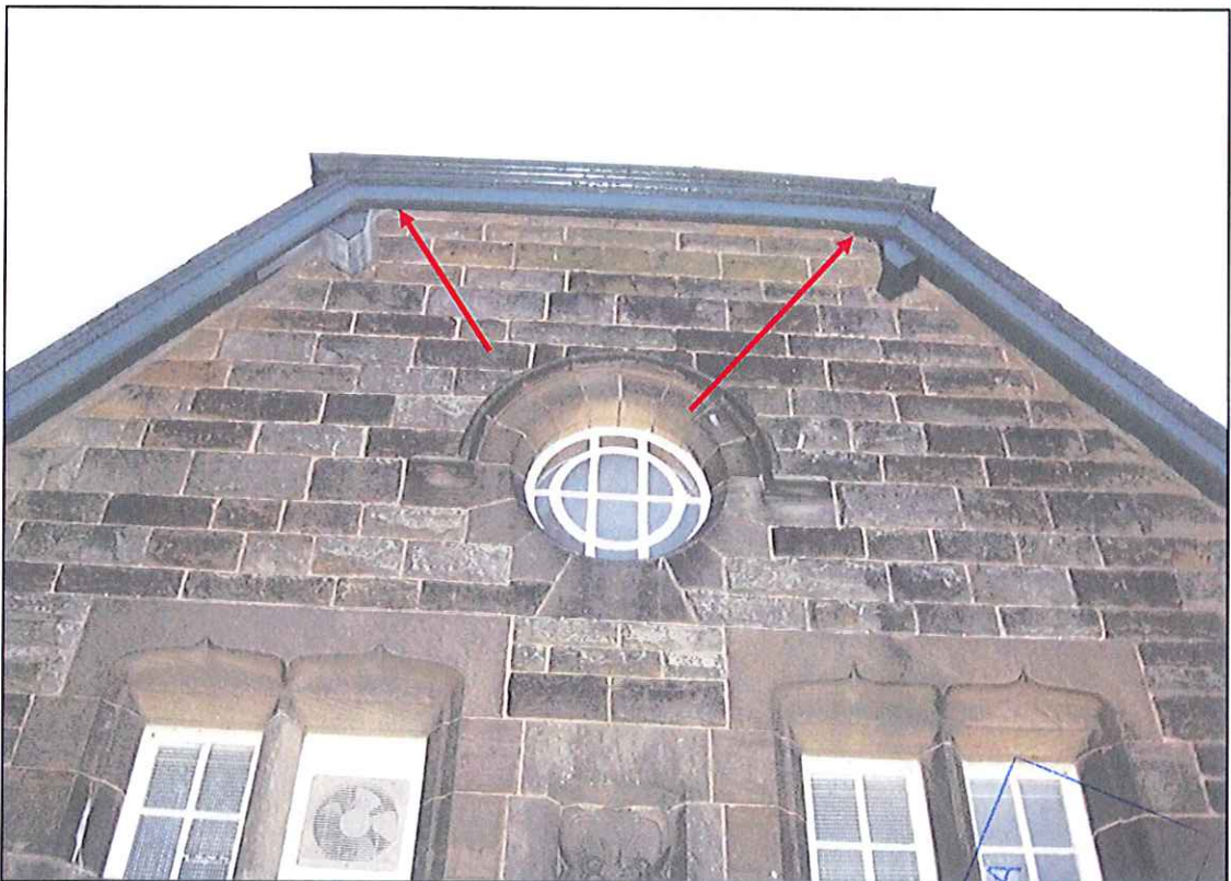
South elevation roosts: Common Pipistrelle to left & Brown long-eared to right
