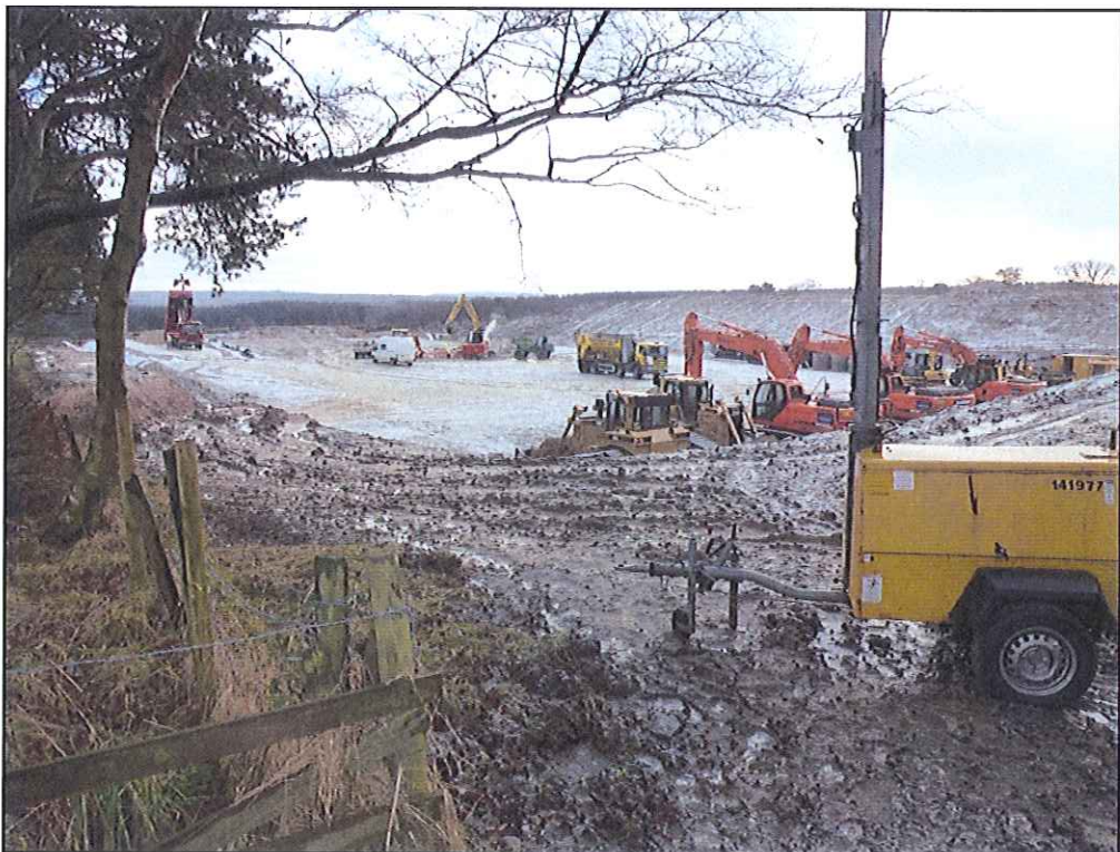
Photograph 1 – Borehole Platform viewed from North-west Corner
