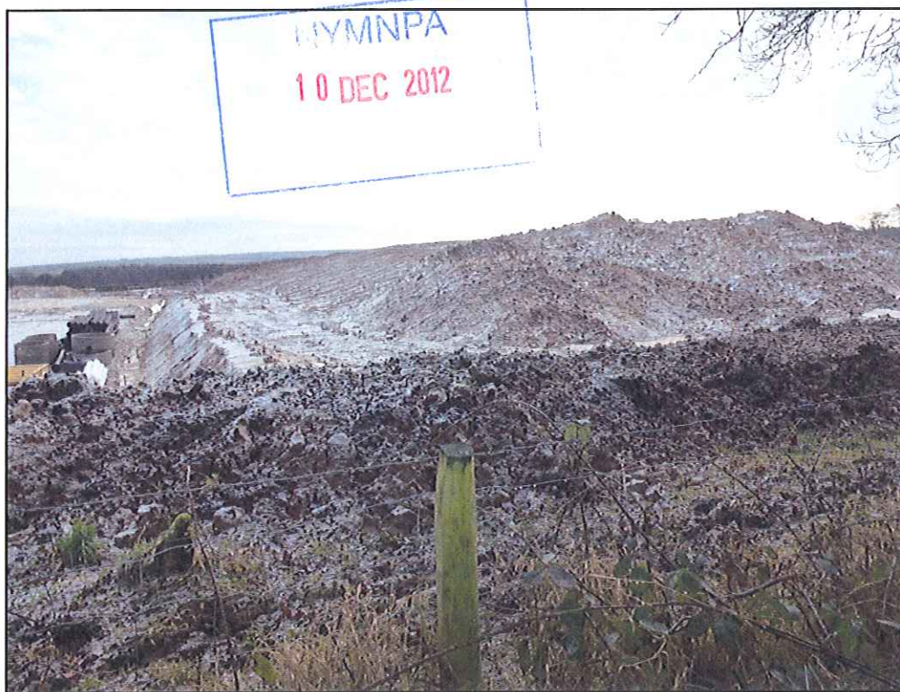
Photograph 3 – Spoil Storage Viewed from Mid-western Boundary
