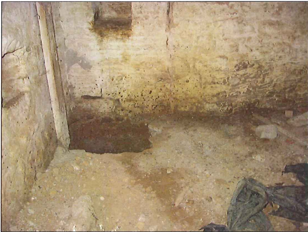
Example of test pit to check foundations
