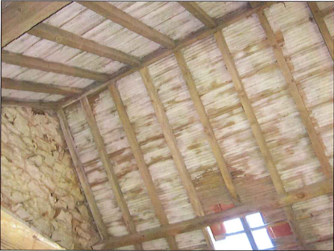
Underside of roof of main barn, 27 February 2013
