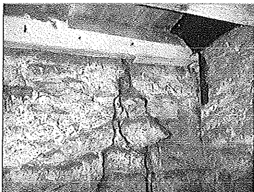
Photo 8 - Deep internal masonry crevice.
