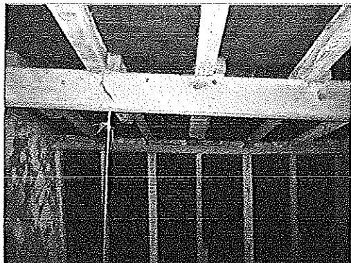
Photo 5 - Thick traditional felt lining to the underside of the roof.
