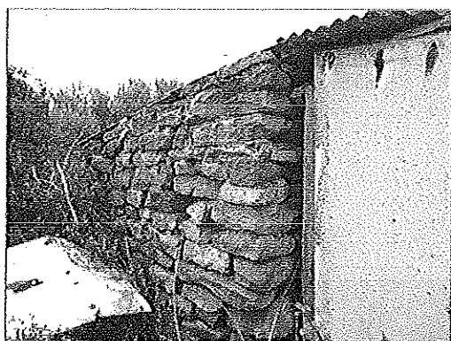
Photo 9 - Dry stone wall section of the attached store.
