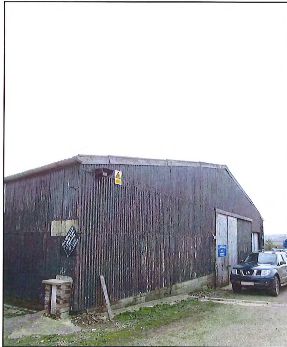
EXISTING SITE PHOTO
